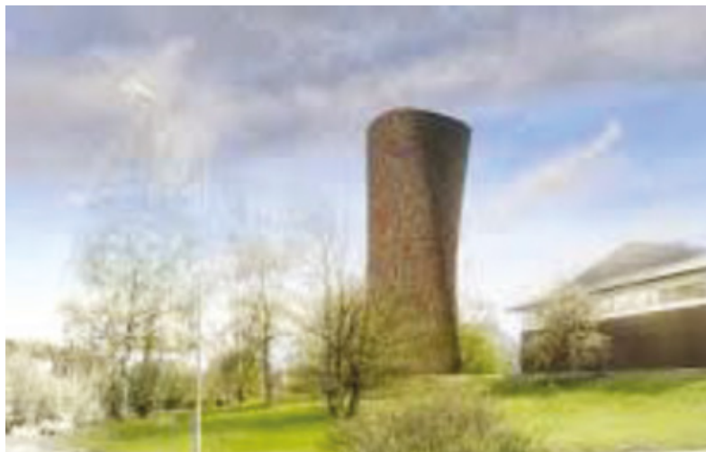
Illustration 31 - Stockholm Northern Link – Shaft for the polluted air exhaust, located upstream tunnel portal
