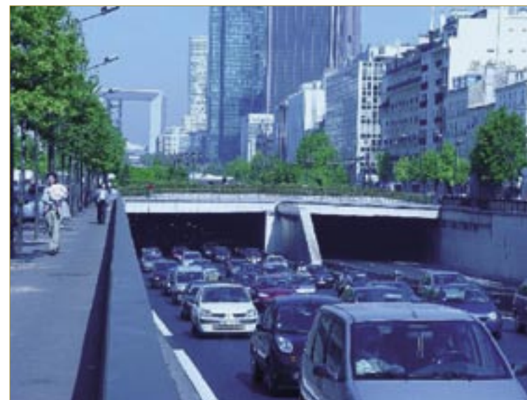
Example of traffic density in an urban tunnel
