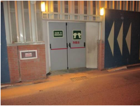
Figure 6 - issue de secours double battant – barre antipanique
