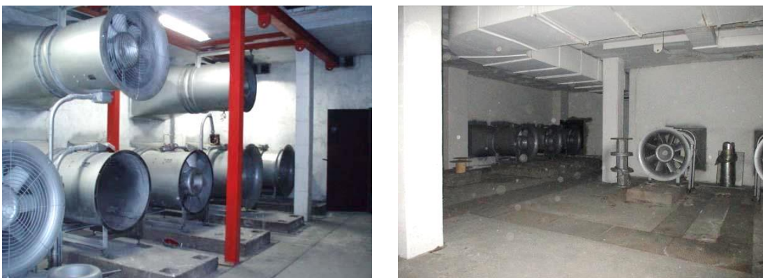
Figure 7 – stations de ventilation
