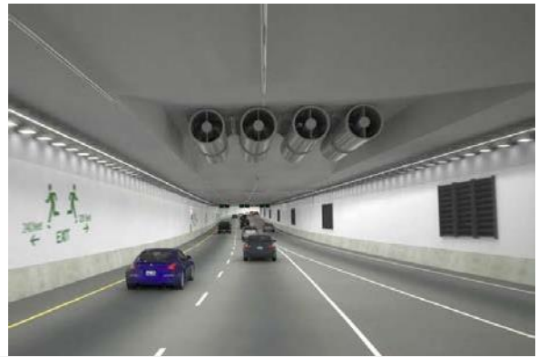
Figure 10 - Tunnel jet fans at portals
