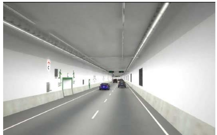
Figure 8 - Overhead electronic signs provide advisory messages.
