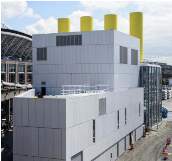
Figure 9 - Tunnel south operation building and two of the four extraction fans
