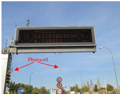
Figure 13 - variable signalling panel (VMS)
