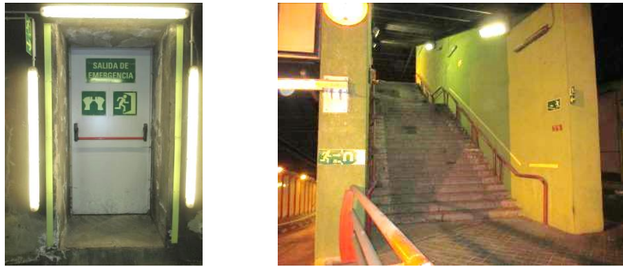
Figure 6 - emergency door and evacuation between the two levels
