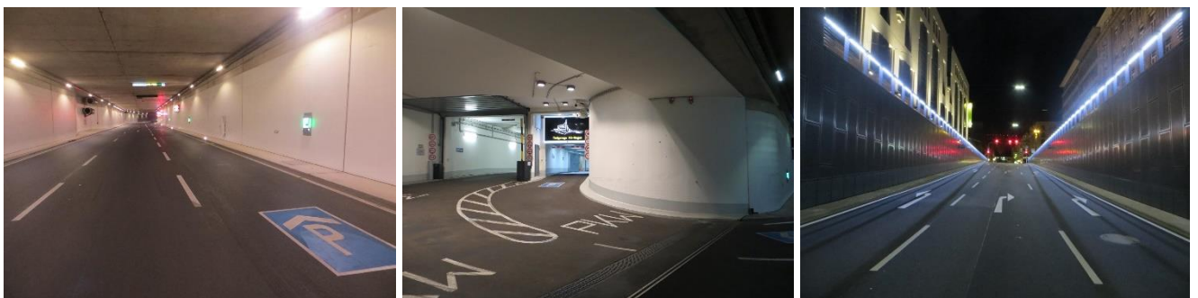
Figure 2 – Tunnel, underground car park and ramp
