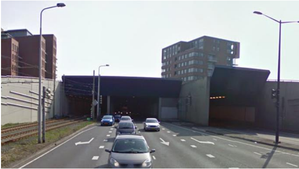
Figure 2: Vliet Tunnel road and rail tubes
