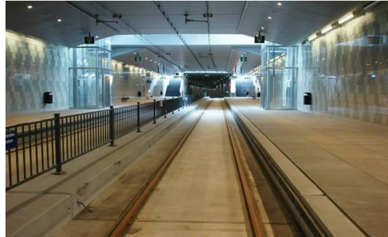
Figure 3: Underground rail station in the Vliet Tunnel
