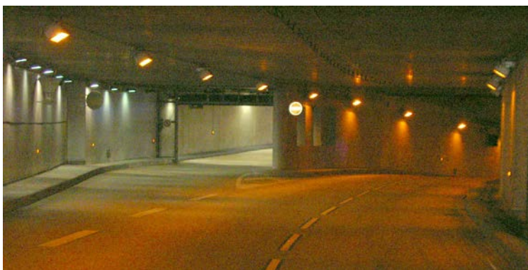
Figure 9 – view of the exit from car park
