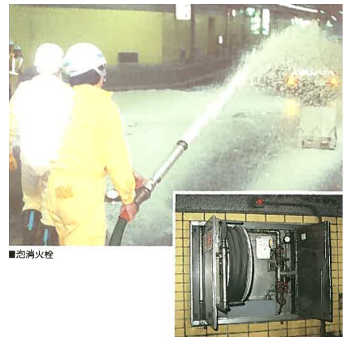
Figure 10 - Foam Fire Hydrant
