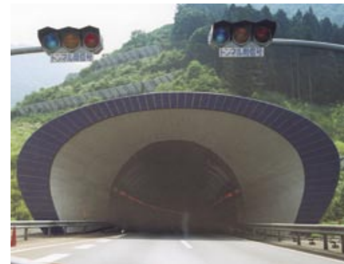
Figure 26: Portal of Kanetsu tunnel in Japan
