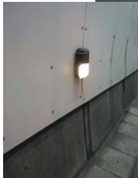
Figure 30: Permanent evacuation lighting used for road guidance in Spanish tunnel
