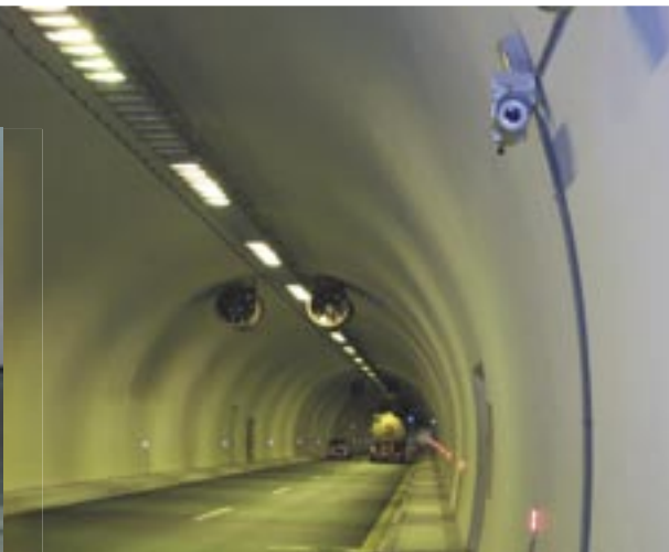
Figure 30: Permanent evacuation lighting used for road guidance in Spanish tunnel
